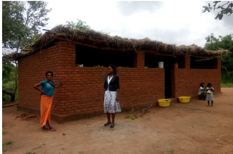
Mkanda Mateyo Primary School has a new school kitchen made possible from the community contribution of molded bricks.
