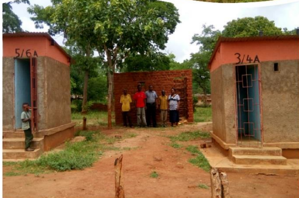
Chigumukire Community School is able to build teacher housing on the school grounds (above) and a girl-friendly washroom (below) thanks to the availability of water and raised awareness.
